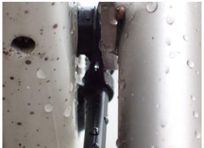
spacers are used to add the needed clearance
